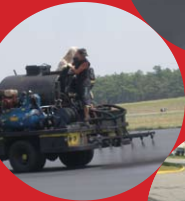
Catch Basin repair
